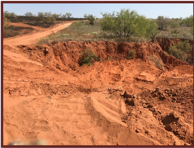
Looking into ravine after dozer removal
